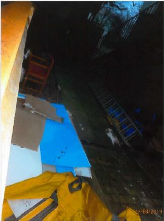
Physical damage and emergency exit
